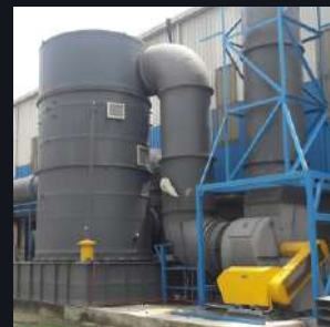
Packed Bed Scrubber for Acid Fumes extraction
